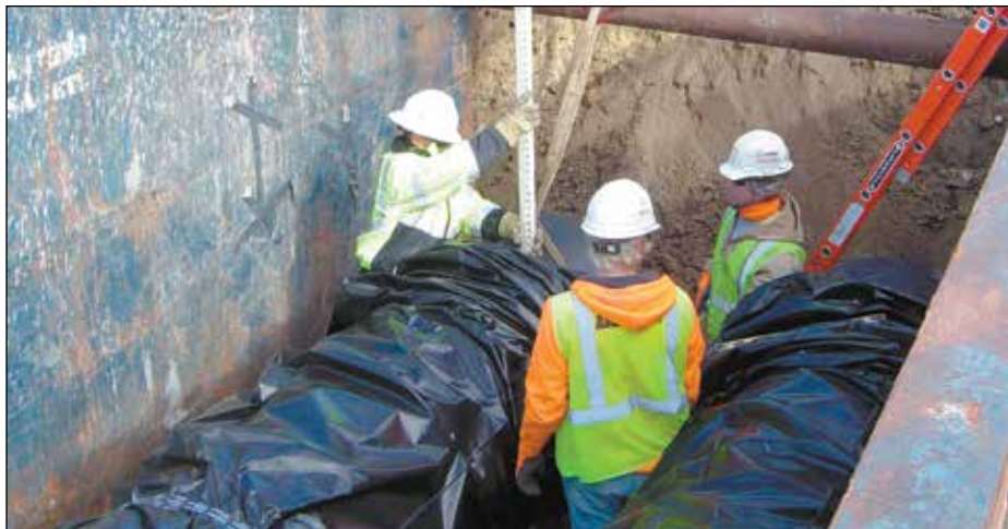
Crews check for elevation while installing the pipe.
