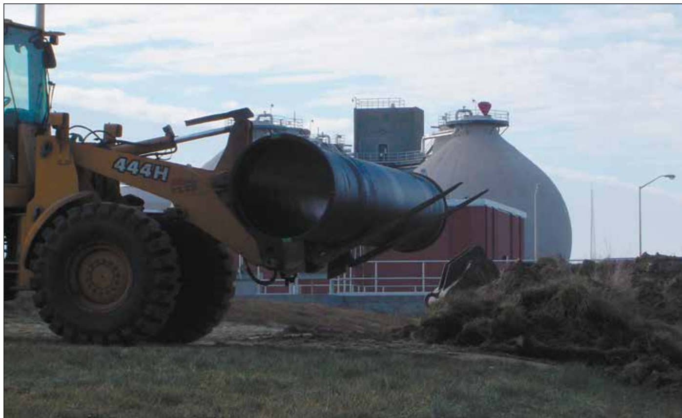
Crews transport ductile iron pipe for installation.
